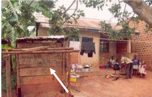
Figure 4: Altered frontal space. The timber shade (foreground) used as a kitchen is a later addition required by a woman. Mbuya. (Photo: Nnaggenda-Musana, 2004).
