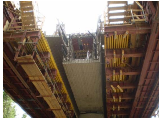
Figure 2: Mobile falsework
