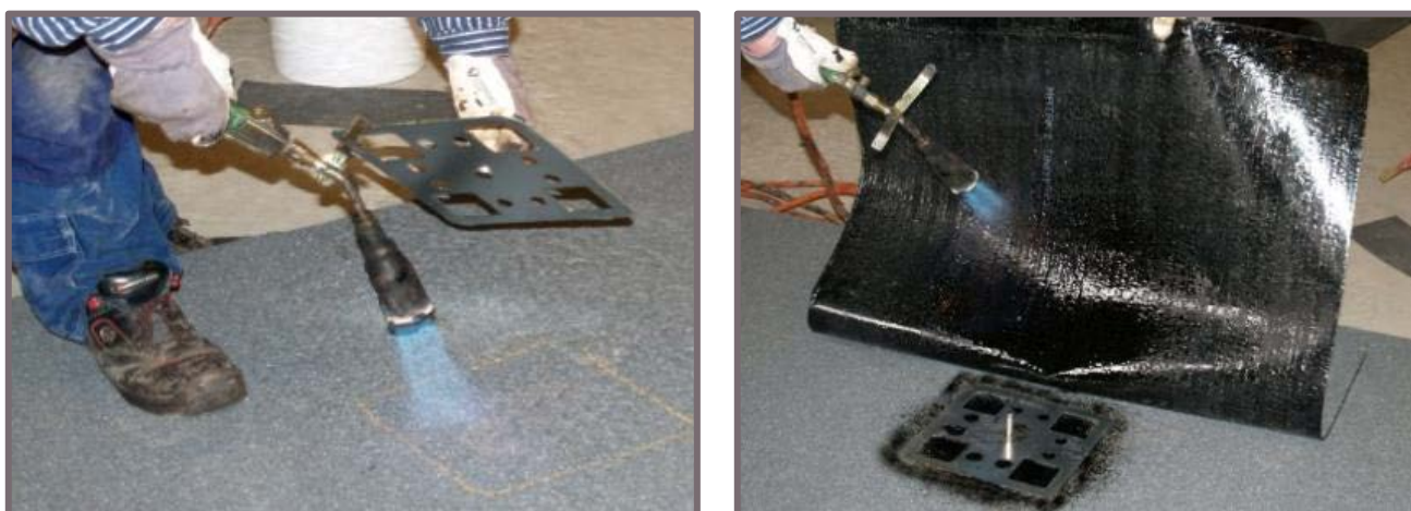
Figure 30 - Installation of a Lifeline roof connection 16
