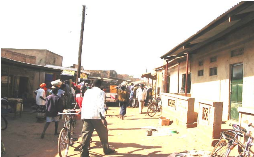
Figure 2: Burnt redbrick, cement wall and iron roof shop.
