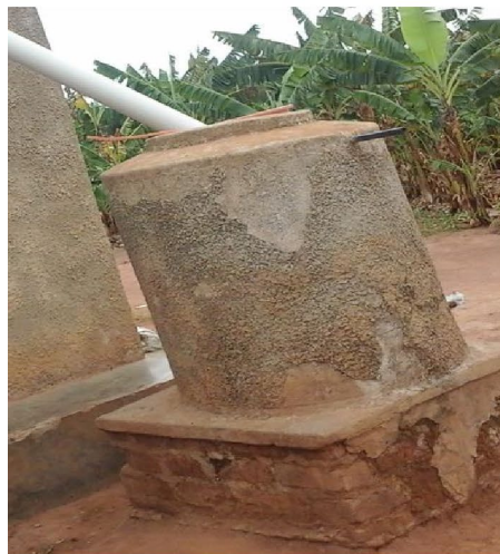
Concrete ferro-cement tank (c)
