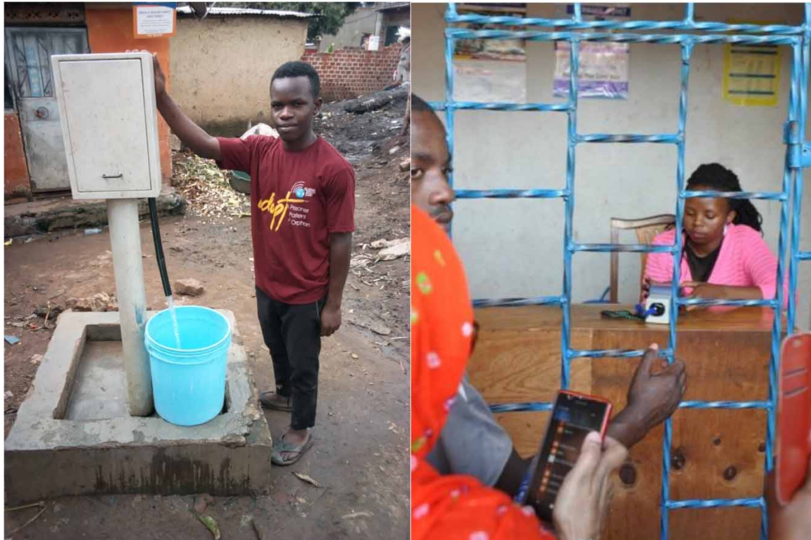
Figure 1 | (a) Prepaid water dispenser and (b) sales point for water credit (consent granted).
