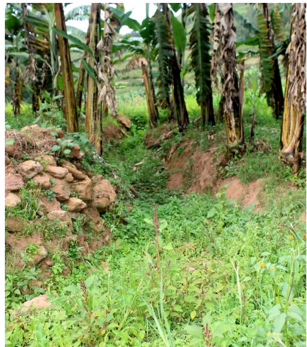
Fig. 12 a, b. Soil, water and land conservation measures to reduce landslide impacts, 2020 (Photo credit; D. Nseka)
