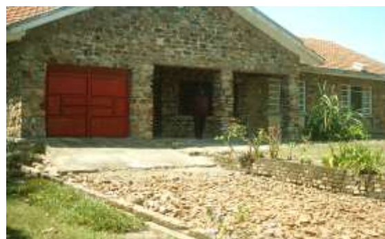
Fig. 4: An example of stone used as a maintenance free building material.
