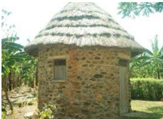
Fig. 3: Use of thatch and stone for a simple dwelling in Mbarara, western Uganda.
