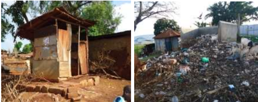
Figure 6: Poor Sanitation facilities in urban poor settlements
