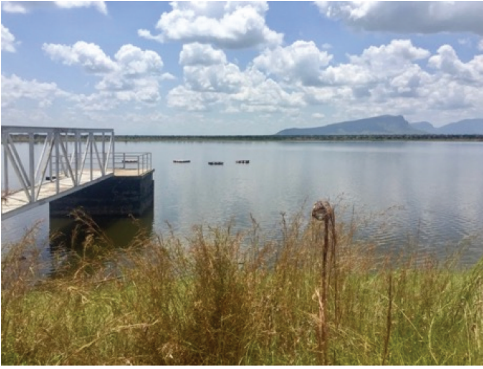
Figure 5. Archet dam, October 2017.
