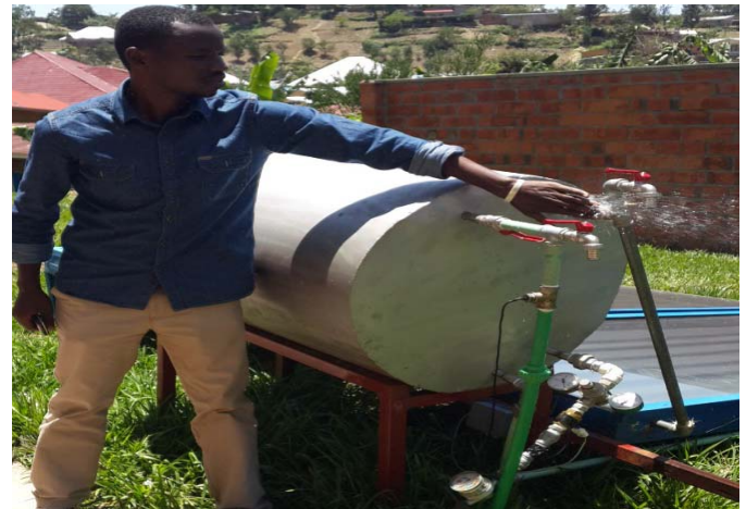
Fig.15.Solar water heater with Smart Meter System
