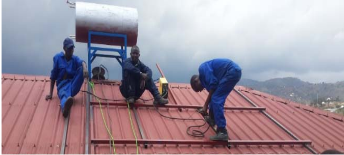
Fig.12.Fixing the solar water heater on the roof of house
