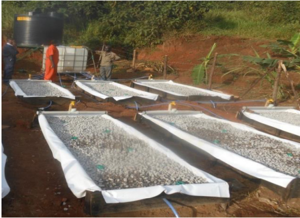
Fig. 3 Construction of collard based bio-filter.
