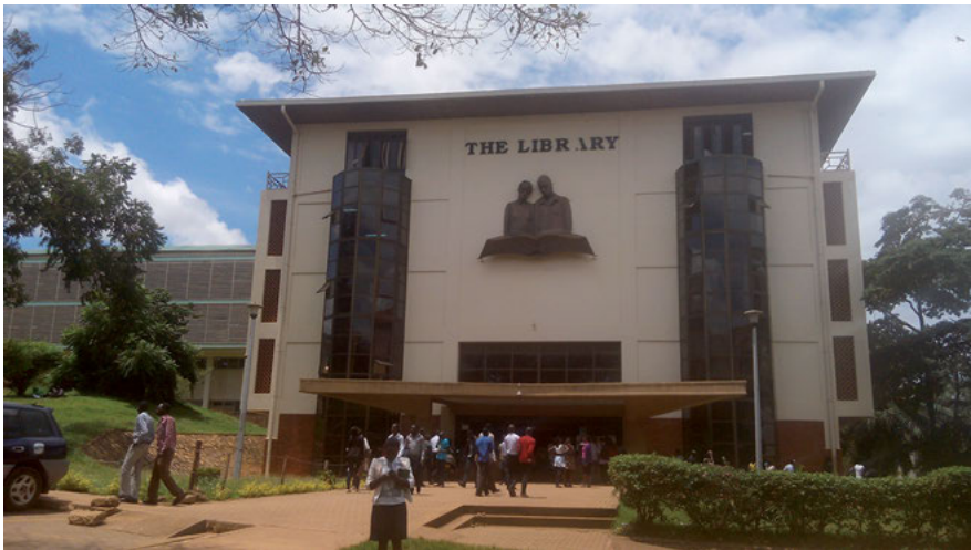
Figure 8.1: The new library building, ready 2012. (Photograph by Makerere University).
