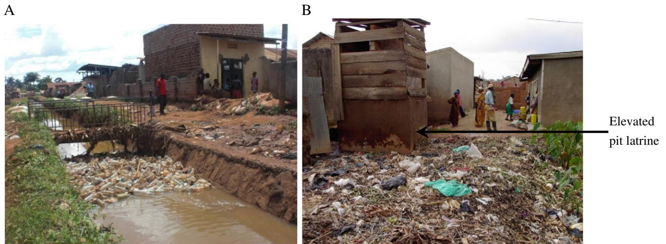
Fig. 6. Photographs illustrating sanitation status in Bwaise III in Kampala (Uganda). (A) Blocked storm water drain and (B) solid waste dump and an elevated pit latrine in the vicinity of a household in a slum area.
