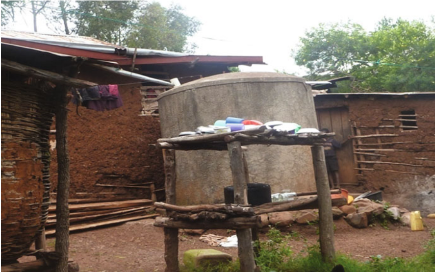
Fig. 23.4 Rain water harvesting in locally constructed water tanks (on small scale, e.g., from rooftops) as drought mitigation measure in Kimbugu village, Isingiro district, Uganda
