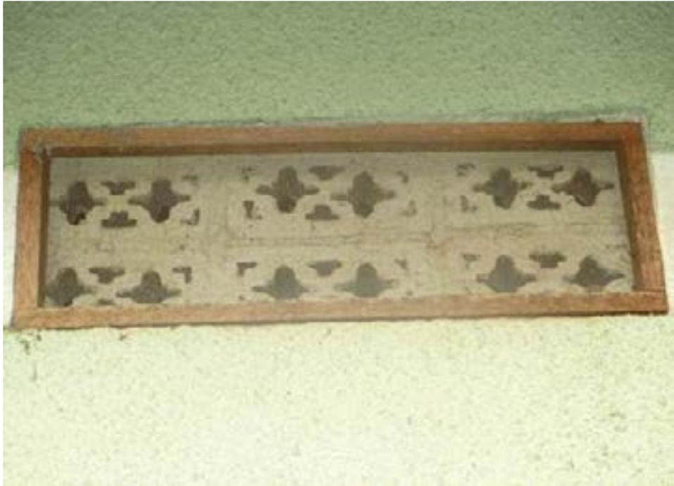
**Figure 2. A ventilator with screening on one of the demonstration houses.**
